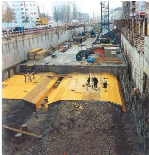
Top-down construction roof formwork
