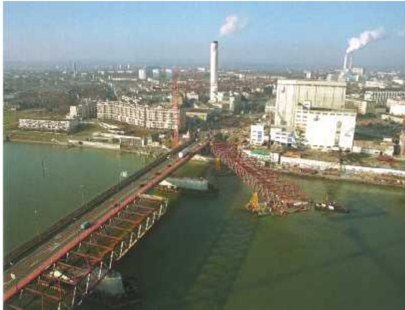
Transportation and Placing of the new steel construction
